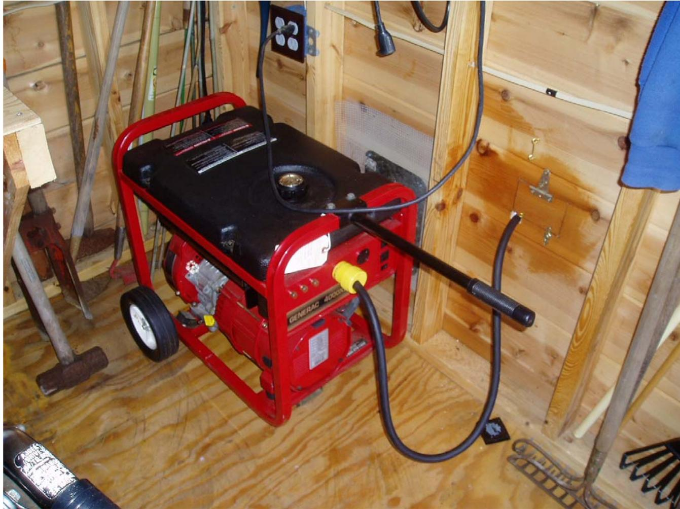
My Generator installation - inside a tool shed - exhaust is Vented outdoors
