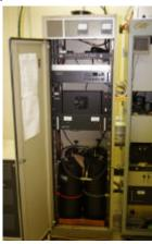
We took all three repeaters down around 10:00 AM and starting tearing out all the pieces. We then followed the new layout diagram Ernie had drawn with a few corrections. The biggest challenge was trying to put both sets of 2 meter duplexers in to one cabinet so the whole assembly was within the cabinets. With a lot of tape measuring and some mechanical acrobatics, we were able to get them in the one cabinet.
